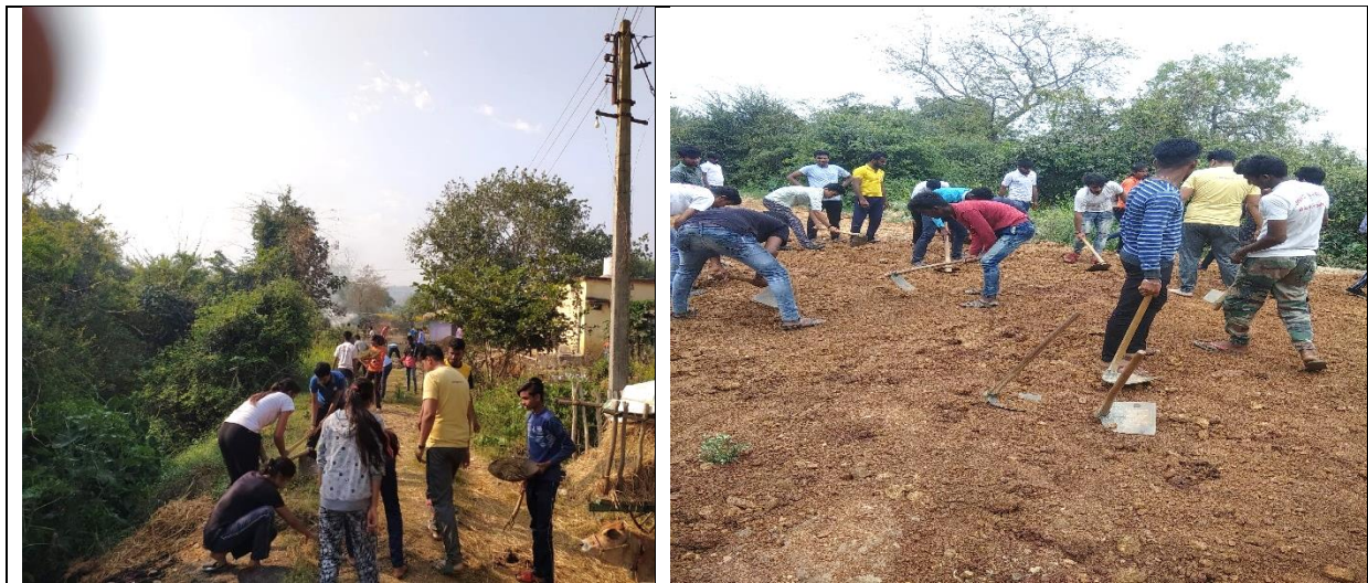
The campers constructed a 300 metres double bypass road
